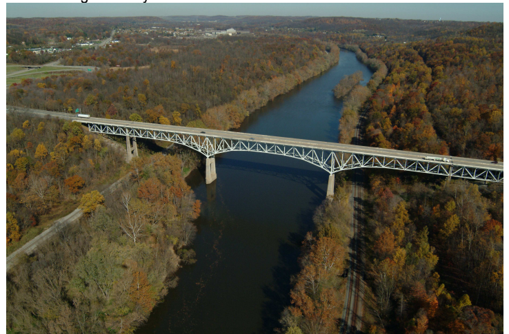
This photo shows an overall view of the existing bridge over Beaver River.
